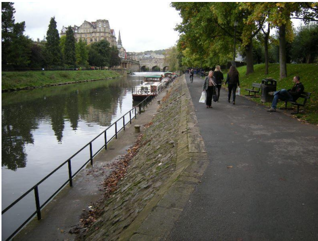
Photo 11: View of moorings below sluiceway/ weir with river at normal level
