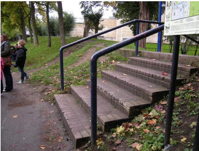
Photo 7: Main entrance with steps and parking in front
