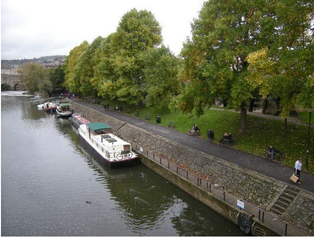
Photo 9: View of moorings below sluiceway/ weir with river at normal level
