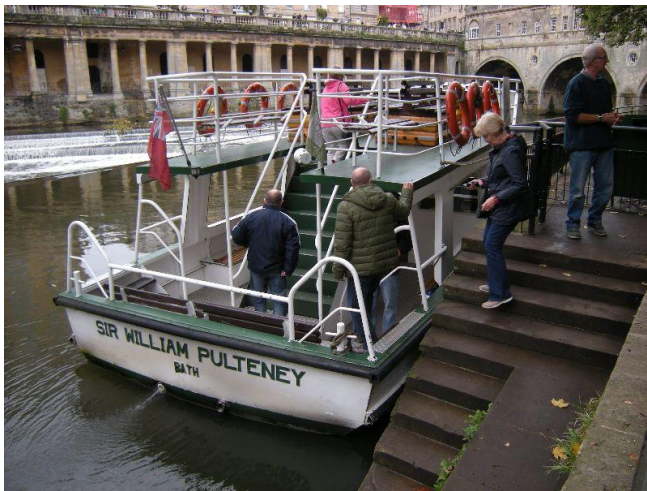
Photo 3 Steps with no handrails down to cruise boat embarkation point
