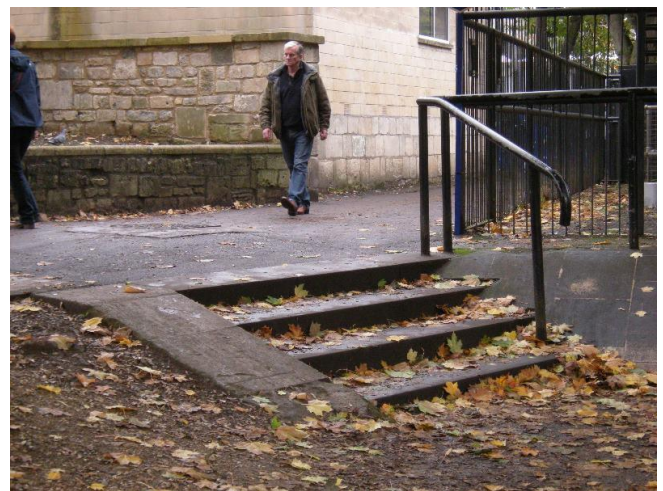
Photo 4 Steps with one handrail near sluice gate
